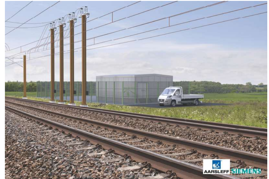
Autotransformerstation
